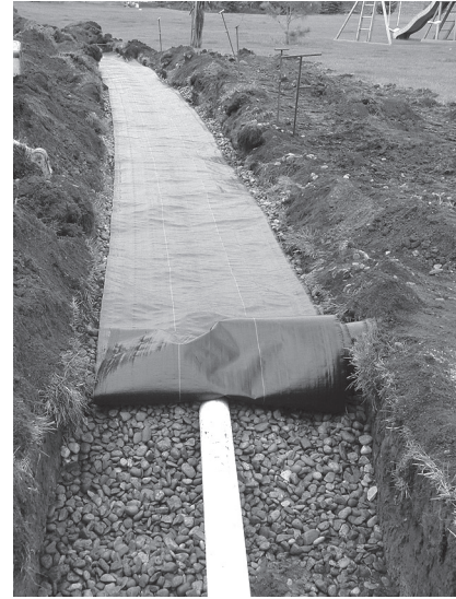
Figure 13. Gravel-filled trench covered with geotextile fabric.
