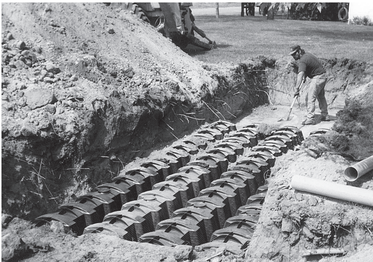
Figure 17. Chamber-type gravelless system being installed on a very small house lot. Normally the chambers would be used in trenches.
